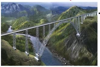
Being constructed to withstand an earthquake of 8 magnitude, this railway bridge is part of the Udhampur-Srinagar-Baramulla rail project. Slated to complete by March 2021 which is 359 metres above the Chenab riverbed, stands 35 metres taller than the iconic Eiffel Tower in Paris.
